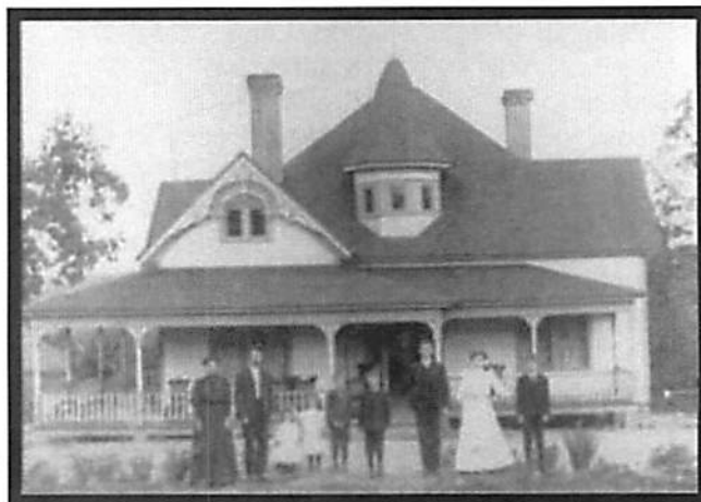
Home of James Madison Garrett and Mary Entrekin Garrett of the Hurricane Community near Six Mile, South Carolina. The house was probably built in the early 1890's. This photograph was made about 1900. It burned in November, 1928, the same year as the Six Mile tornado (March, 1928). Left to Right: Mary Entrekin Garrett, James Madison Garrett, Lois Garrett, Leola Garrett, John Perry Garrett, Ralph Wyatt Garrett, William Calvin Garrett, Elizabeth Emily Garrett, and James Albert Garrett. (Photo courtesy of Tandy Martin "Tom" Jones, III)
